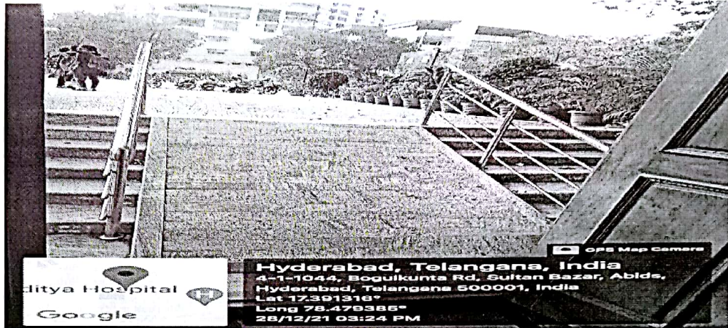
Ramp at E Block
